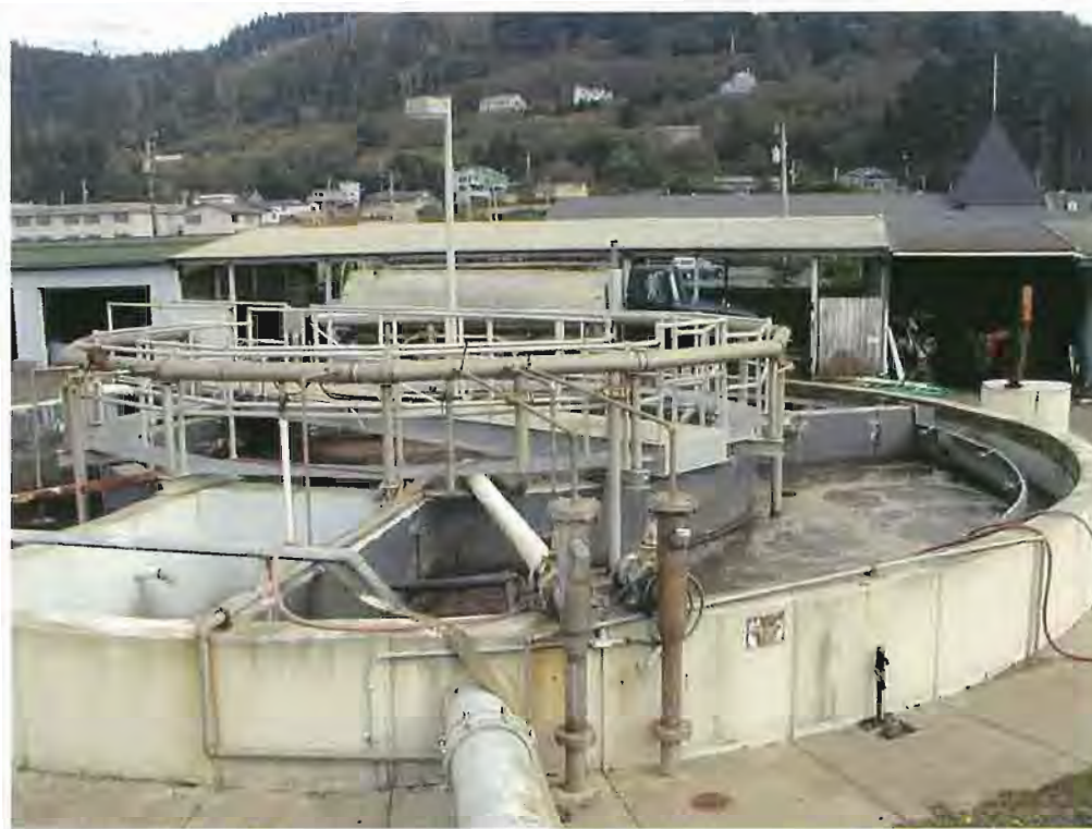
FIGURE 3.3.1 YACHATS WWTP, AERATION BASINS & DIGESTERS
