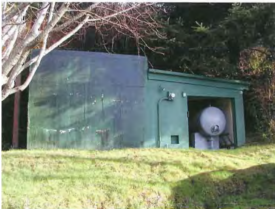
10,000 Gal. Concrete Reservoir and 1,000 Gal. Pressure Tank – Upper Tank
