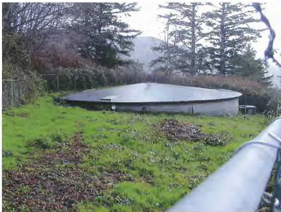
200,000 Gal. Concrete Reservoir – Round Tank
